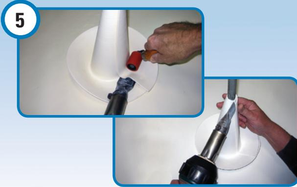
5. Tack weld the inside of the overlap where the base transitions to the collar – then tack the top of the collar snug to the penetration.
