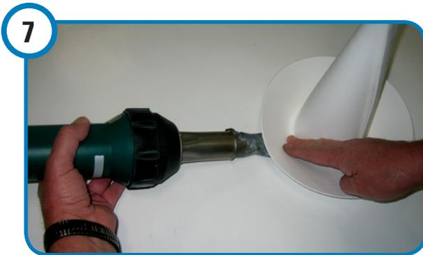
7. Weld the base flange. The flange may funnel up slightly but is easily formed flat when heated during the welding process.
