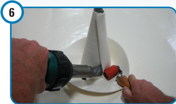
6. Weld the vertical seam of the collar first, using the penetration as a back stop for welding compression.
