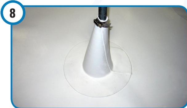
8. Finish welding the base, probe all welding to ensure continuity and finish off the detail by installing the supplied stainless steel worm gear clam at the top of the flashing and seal with a tooled bead of FTR 101 Sealant.
