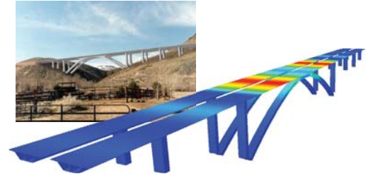
Galena Creek Bridge (Nevada, USA)
