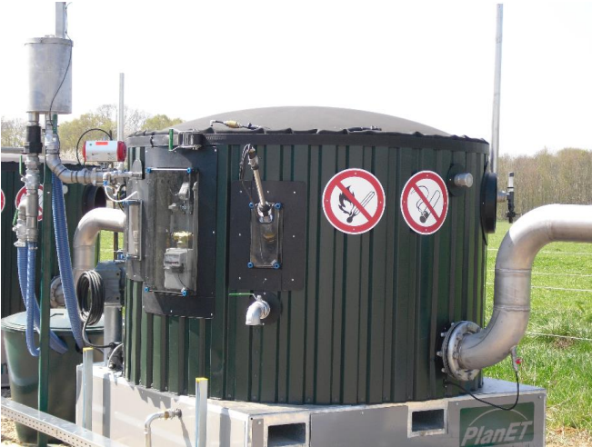
Anaerobic digesters
