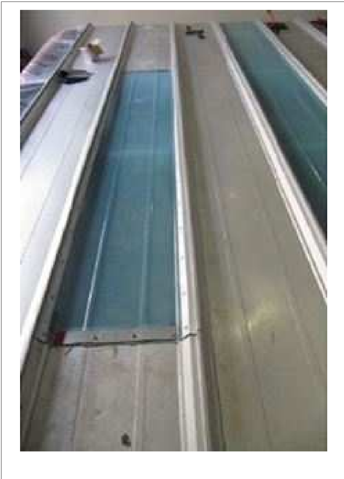
Fig. 3. Skylight for use in SSR panels
