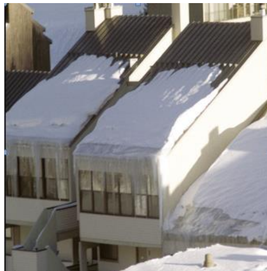
Figure 6B: Ice dams create unintentional snow retention
