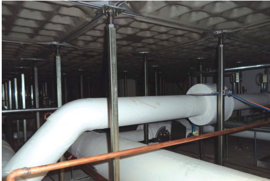
Figure 1: Chilled water pipe serving the data center is shown. Branch piping to computer room air handling units and condensate piping is also visible. Courtesy: ESD
