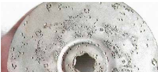
Pitting corrosion of EN 1.4401 (AISI 316)
