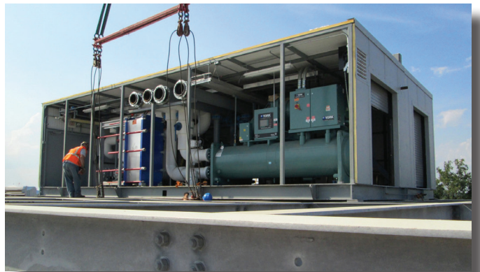
FIGURE 1. Two (2) chiller, one-section complete packaged chiller plant
