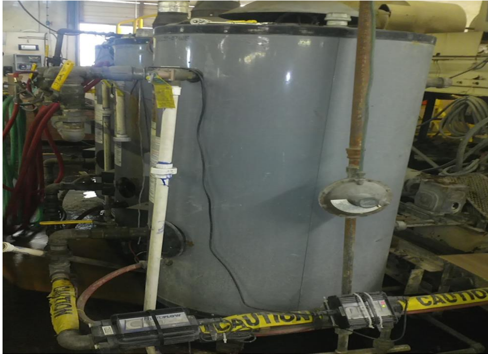
10-24-11 -HydroFLOW C-60 Unit installed on 3 Industrial Water Heaters
