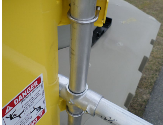
U-Bolt connection to vertical handrail pipe.
