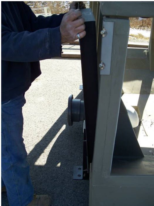
Set the louver in the opening.
