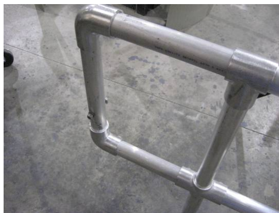
Match drill the ladder to the handrail.
