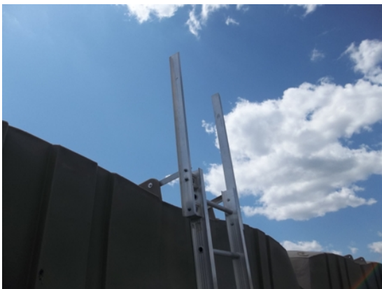
Bolt the ladder into the lifting lug.
