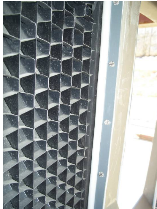
From inside the sump, confirm the louver is against the gasket. Adjust the gasket as needed.
