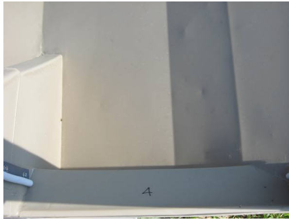
Louvers are numbered with the top identified. Each opening on the sump has a matching louver number.
