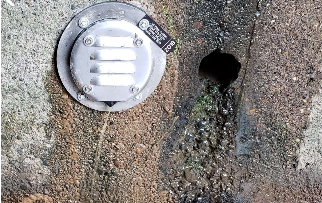
Figure 3 – Existing Weep Hole with Abraded Concrete
