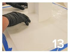
13. Apply evenly spread Forti-Lock Liquid Flashing resin base coat onto the horizontal surface at specified application rate (approx. 50 wet mils). Place the horizontal Forti-Lock Reinforcing Fleece pieces.
