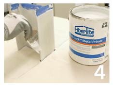
4. Mask penetration to a minimum of ½ inch (1.3 cm)beyond intended material application area. Prime metal surfaces with Forti-Lock Metal Primer per application rate of approximately 250 ft² (23.2 m²) per gallon. Allow primer to dry a minimum of 6 hours.
