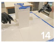
14. Apply a uniform topcoat of Forti-Lock Liquid Flashing resin fully saturating the fleece (Approx. 25 wet mils). Avoid folds, wrinkles or air bubbles.
