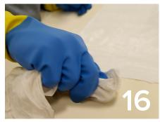
16. Clean up excess resin outside the flashing area by wiping with FiberTite Seam Cleaner and a clean cloth only while flashing is still wet.
