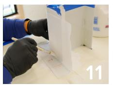
11. After mixing, apply resin to clean and prepared substrate at the required consumption rate, using ½-inch nap rollers and disposable brushes. Apply base coat of catalyzed Forti-Lock resin onto the vertical substrate and immediately apply the Forti-Lock Fleece reinforcement into the wet base. Continue around entire penetration, covering vertical surfaces with precut fleece.
