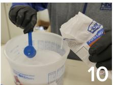
10. Add pre-measured catalyst to the resin component, stir with stir stick for 2 minutes before applying to substrate. Forti-Lock Catalyst Powder addition is based on the weight of resin being used and ambient temperature.
