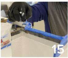
15. After the flashing is fully saturated and complete, remove the tape while the resin is wet.
