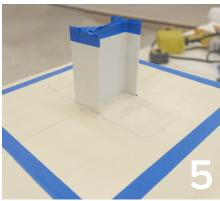
5. Apply masking tape at the top edge termination and on the FiberTite membrane. Mask membrane area a minimum of 8 inches (20.3 cm) horizontally beyond the base of the penetration and 8 (20.3 cm) inches vertically on to the penetration (½ inch below primer line).
