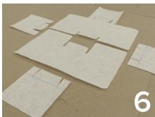
6. Pre-cut Forti-Lock Reinforcing Fleece as required prior to mixing and applying with Forti-Lock resin. The Forti-Lock Fleece should conform to penetrations being flashed. See detail FTR-FL4.
