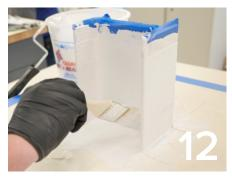
12. Apply a uniform topcoat of Forti-Lock Liquid Flashing resin fully saturating the fleece. (Approx. 25 wet mils). Avoid folds, wrinkles or air bubbles.
