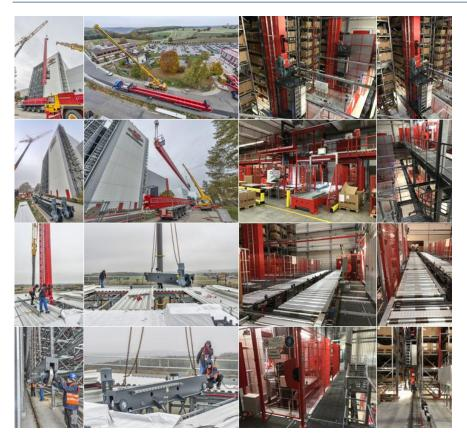
Image caption: Kardex Mlog built, delivered, and installed four MSingle B 1200 storage and retrieval machines (SRMs) with aisle equipment and automatic control for Adolf Würth GmbH & Co. KG. They integrated the SRMs across three floors in Würth's existing plant.
