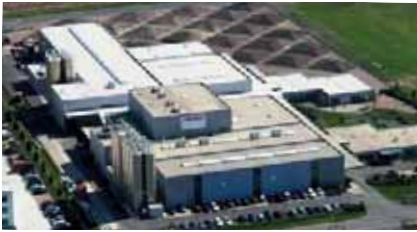
Production centre for STARstrap™ strapping in Germany
