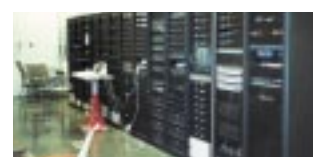
The neat central rack room
