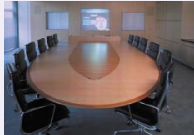
One of six presentation rooms at the Cisco Executive Briefing Center equipped and serviced by Electrosonic. The center screen is also an interactive board, using a Smart Technologies™ SMART Board 580; the flanking side screens are electronic whiteboards, so images from all three can be captured and saved as computer files. Each room has an AMX Axcnt 3 room controller with an LCD touch screen as the user control. The table is arranged so that any participant can connect a laptop computer into the system.
