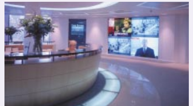
A media wall showing a mixture of PC graphics, DVD video and satellite television is a prominent feature of the reception area at the Cisco Executive Briefing Center. The display uses Electrosonic's VECTOR™ image processing and Toshiba projection "cubes".
