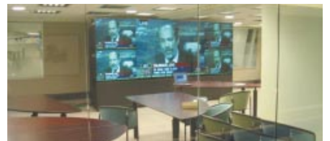
The videowall used in Star TV's Mumbai studios is made up of an array of 7x3 screens to achieve a display 24ft x 7.75ft (7.3m x 2.35m). It uses a frame construction developed by Electrosonic Systems Inc for permanent installations. Each screen module is 53 inch diagonal, and the projectors used are Pioneer videowall "engines". Photo by Alec Wood.
