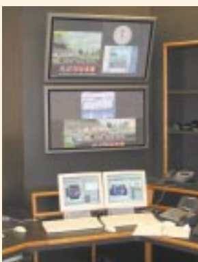
A corner of the control room, showing the C-THROUGH programming of the two main displays.
