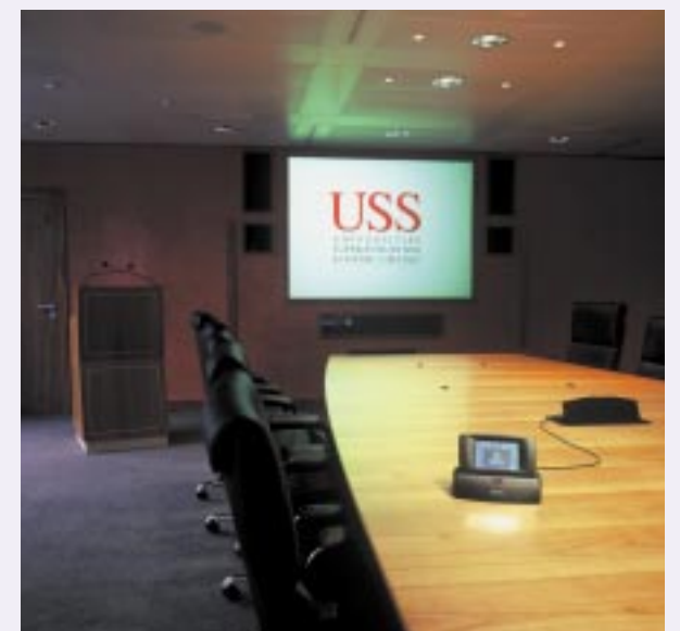
The USS Boardroom in the City of London has extensive conferencing facilities. The bright image is provided by a combination of Barco IQ G300 projector, DNP rear projection screen and custom built mirror projection stand. Installation by Electrosonic Ltd.
