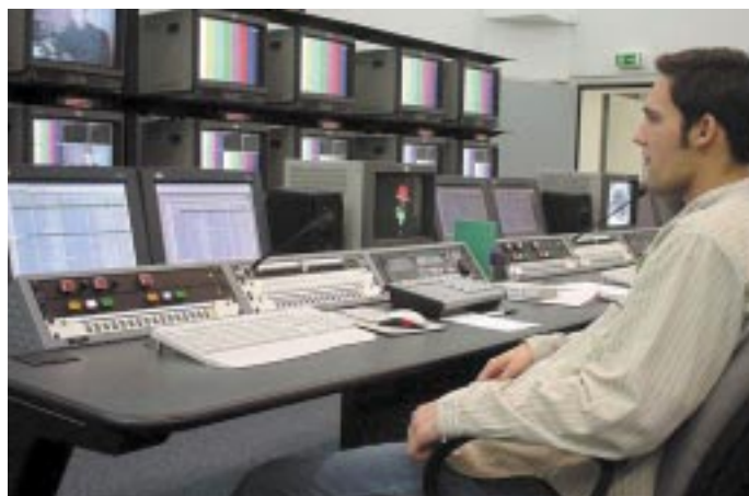
Qualitron engineer professional broadcast installations, like this automated playout system for YLE. (Finnish Broadcasting).
