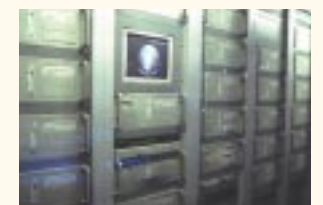
The central equipment is housed in eight rack cabinets within a room that is externally themed to be part of the exhibition. Visitors can see the equipment, normally dramatically lit, through "portholes". All AV exhibits are under Electrosonic ESCAN™ monitoring and control. Daily operation is from a touchscreen that can start and stop the whole exhibition, and can modify the regime for special events.
