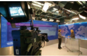
The TV interview studio includes a videowall that uses VECTOR™ processing. While the TV studio equipment was installed by others, Electrosonic provides the on-site support service for it.
