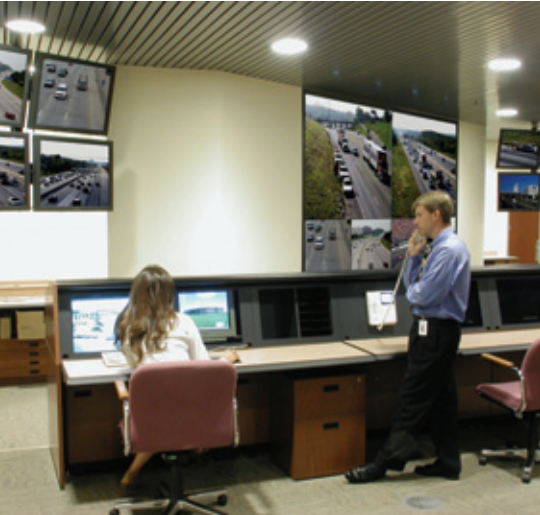
The Kansas City Scout Operations Center in Lee's Summit, MO, monitors 75 miles of freeway in Metropolitan Kansas City. Electrosonic VDS delivered the display system which consists of eight Pioneer 50 inch plasma displays and 12 Clarity 52 inch DLP™ cubes. The cubes receive both direct images and the output of a VECTOR processor.
