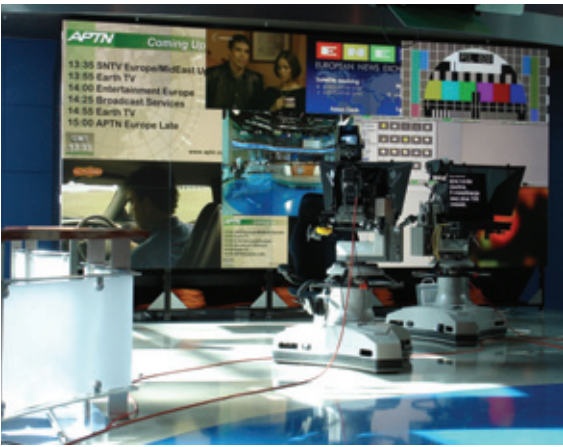
Channel 4 News in the UK broadcasts from a studio within the ITN building in London. It has recently upgraded its set with a 3 x 2 videowall, this time using Barco 67inch XGA cubes. Once again VECTOR's all-digital variant of SDI in and DVI/XGA out is used. However, in this case configuration control is by Electrosonic's COMMANDER™ software. While this has less flexibility than C-THROUGH, it can be easier to use if only a few standard configurations are required.
