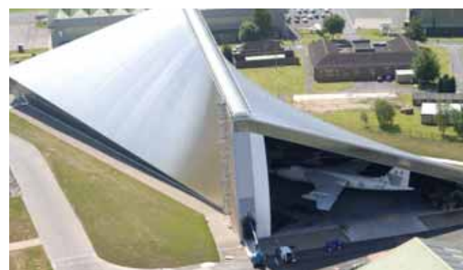
The Cold War Museum at RAF Cosford. The photo was taken when the exhibits were being moved in, the open side is now covered in.
