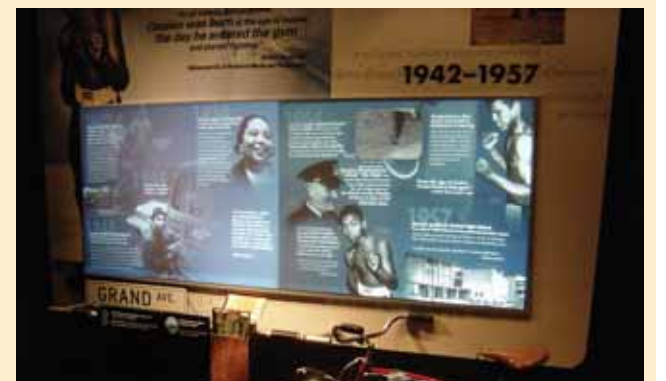
One of the time line interactive exhibits. The four exhibits each use a twin rear screen arrangement using short throw projectors. In this one the interactive input is by touching the bicycle seat – the bicycle was stolen from Ali when he was 12.
