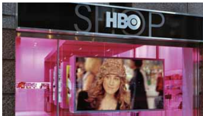
The HBO Shop from the street. At the front, the 4mm LED display, behind it the three vitrines with plasma displays, and to the left a 12inch high LED banner display.
