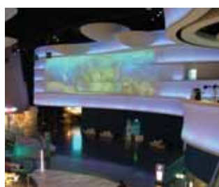
The AV systems at Georgia Aquarium are supported by an Electrosonic service contract.
