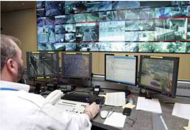
The display can show up to 72 simultaneous CCTV images and six RGB images.
