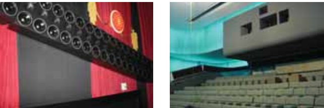
Close up of the loudspeaker array (left). View of the Peltz Theater taken during installation of the Iosono system (right).
