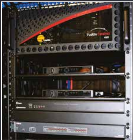
Photographs (left): • One of the video walls based on rear projection cubes. • The video wall source racks contain computer and video sources and a Jupiter Systems Fusion Catalyst processor.
