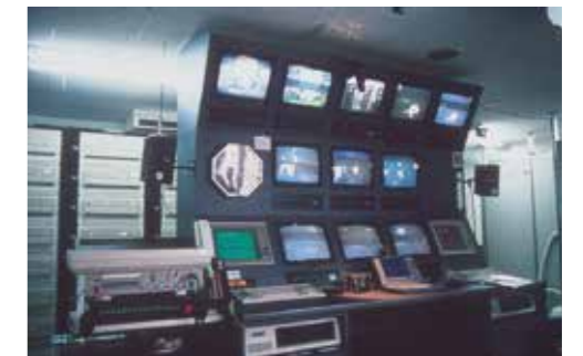
The control console for the Gas Pavilion at EXPO '90
