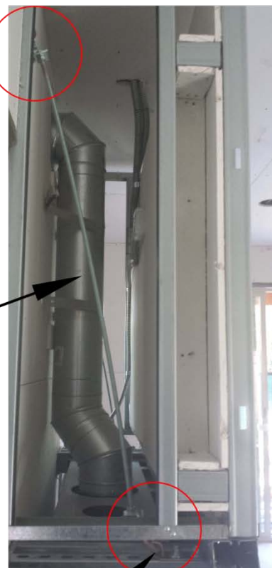
CONNECTION POINT FOR 3/4" ALL THREAD ROD TO HEADER
