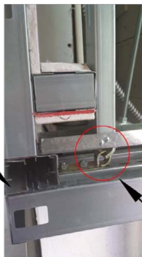
CONTINUOUS BOX HEADER SIDE VIEWS
