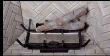
B. Place #1 log on the back of the burner against the grate with "Y" end pointing towards the right.
