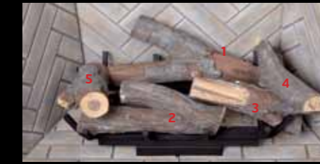
F. Place #5 log so that the front end with the knot is resting on top of #2 log and the back side is on the grate.
