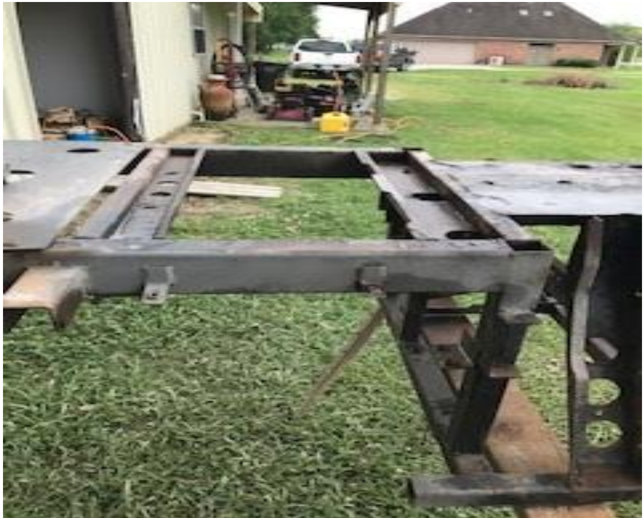
Wet abrasive vapor blast with Corr-Ze 100™
