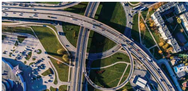
TRAFFIC MONITORING AND MANAGEMENT
