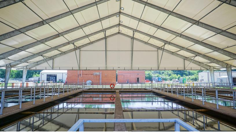
Before making a purchase, the RWRA investigated several options for covering the tanks – including using two separate covers or several types of buildings. "One of the considerations we had was resistance to a highly corrosive water treatment environment," said Cernius. "There's high hydrogen sulfide, so metal quickly degrades."
