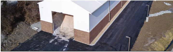
Unlike metal buildings, fabric-roofed structures are inherently resistant to corrosion, making them ideal for salt or fertilizer storage.
