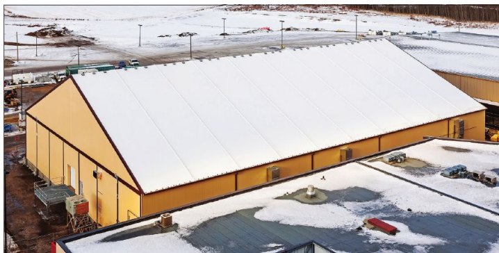
Fabric roofs provide high solar reflectance and thermally non-conductive properties while offering a degree of translucency for natural daylighting.
