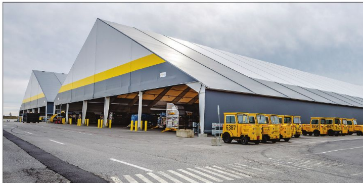
I-beam engineering allows fabric buildings to be specified to exact custom dimensions, including offset peaks and variable column heights.
