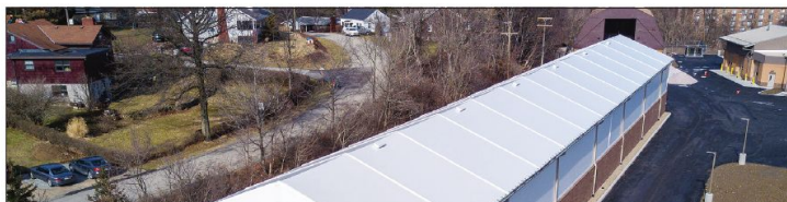
Fabric roofs provide high solar reflectance and thermally non-conductive properties while offering a degree of translucency for natural daylighting.
