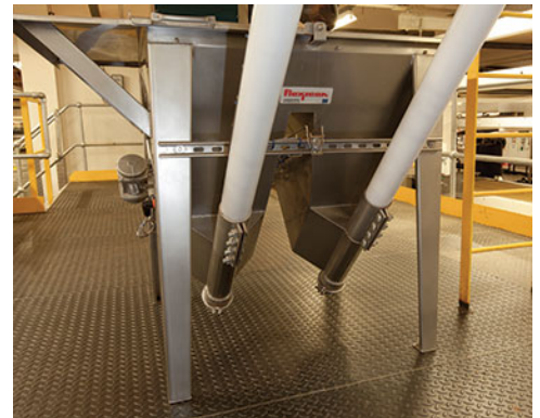
Two types of cocoa powder are emptied into the twin hopper while dust is removed by vacuum. The two flexible screw conveyors move each powder, alternately, to the mixer.
