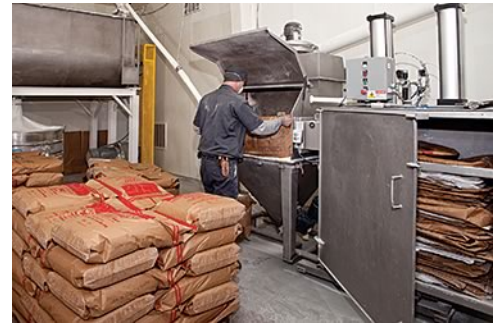
By blending in-house, Franklin Farms East can meet increased demand and expand its product line. The flexible screw conveyor transports minor ingredients being emptied at the bag dump station to the blender in background.
