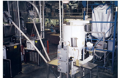
Bulk bag weigh batch discharger (right) feeds weighed batches of cornmeal into vertical blender. Moistened cornmeal flowing into floor hopper at left of blender is fed to two extruder surge hoppers by two Flexicon flexible screw conveyors.
