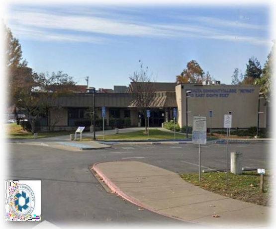
Peralta Community College District Office
