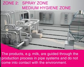
The floor is cleaned with cleaning agents, the products should be insensitive to splash water (corrosion), as well as to chemical vapors that can be generated during cleaning.
