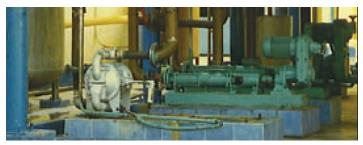
Additional benefits of SANDPIPER HDF pumps compared to Progressive Cavity pumps is the smaller footprint and ease of installation
