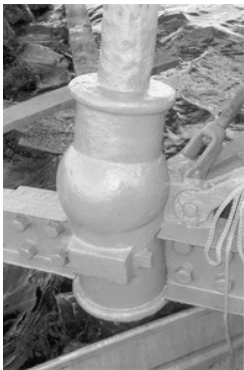
Cast iron coupling at Thomas Point Lighthouse
