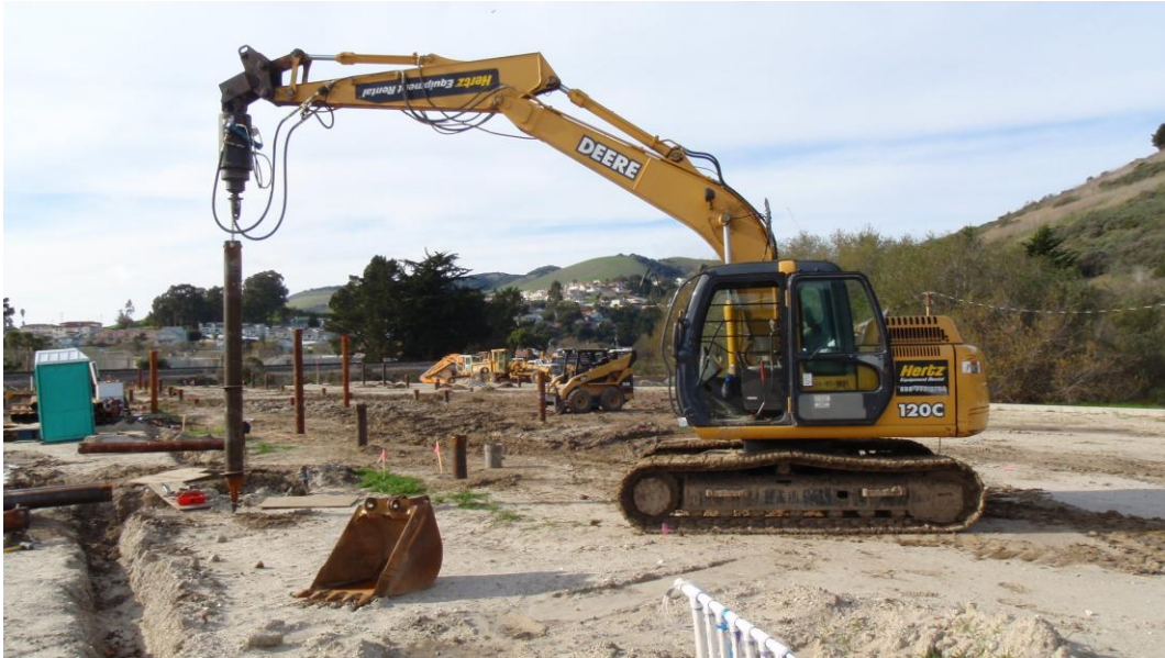
New construction with P8
