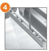
Slide rollers into shoe, secure with set screws and install end cap.
