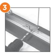
Drill a 1/4" hole in the back shoe for the plunger lock. Screw secure clip onto bottom track between back shoe and front shoe.
