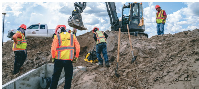
Moving forward, Lane plans to integrate other SYNCHRO applications to facilitate collaboration and overall management and development.
